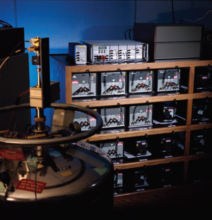
10 V working standards of voltage in the Fluke standards laboratory in Everett, Washington USA.
